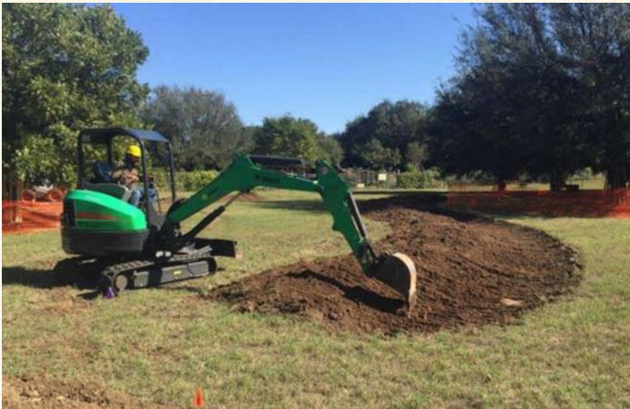
Contour-swales installed will boost rainwater infiltration. Source: Drought Proof Texas at Austin's Festival Beach Food Forest.
